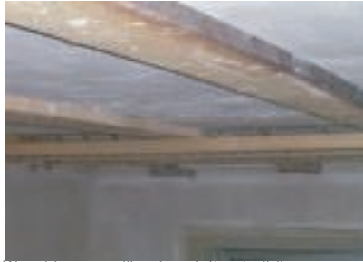
Wood beam ceiling in existing building
