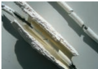
Function maintenance cable with insulating ash layer
