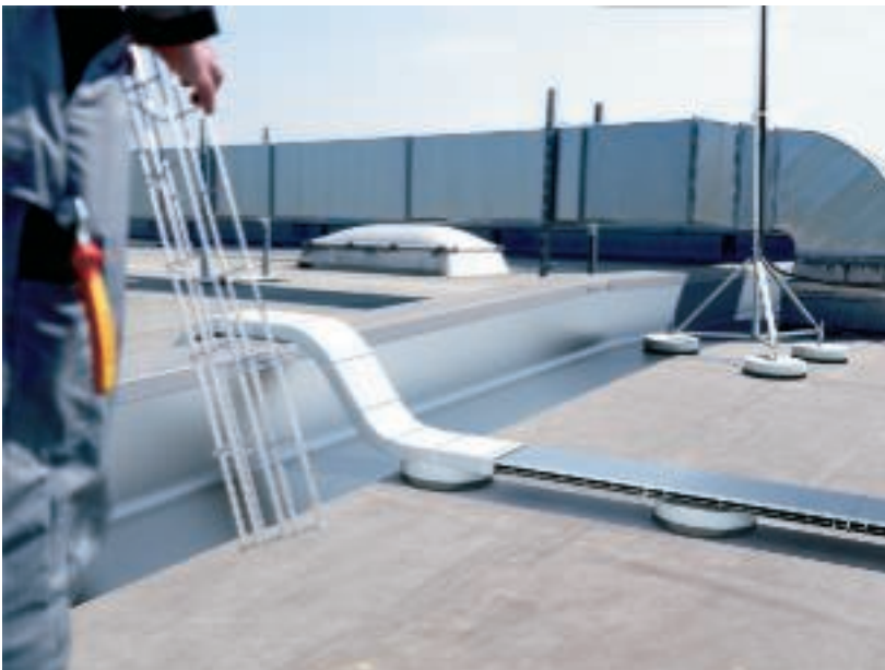
Protected bridging of the fire wall using a fire protection bandage
