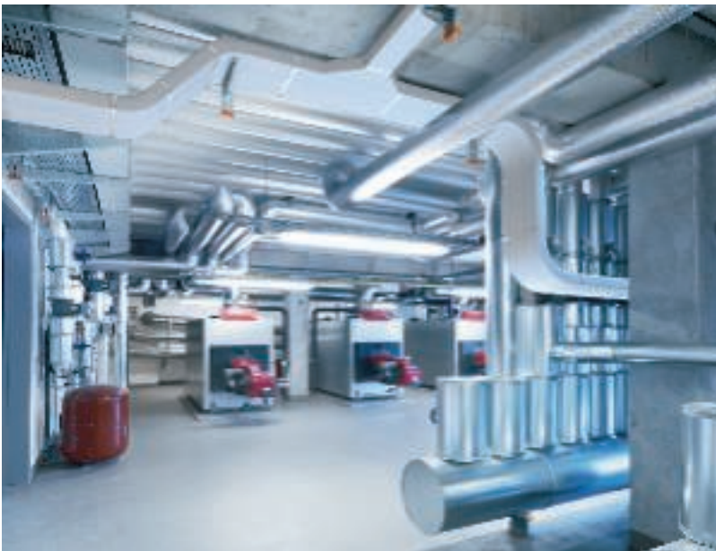
Industrial use of cable bandages
